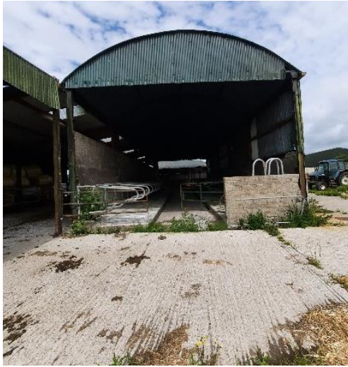
Plate 4-7 Long cow cubicle shed and yard, open on both sides
