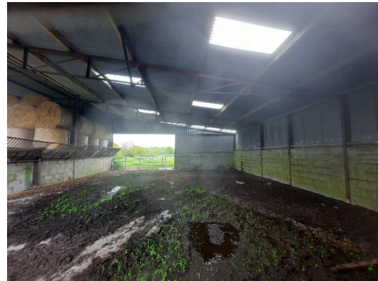
Plate 4-4 Interior hay barn and cow shed with light penetration
