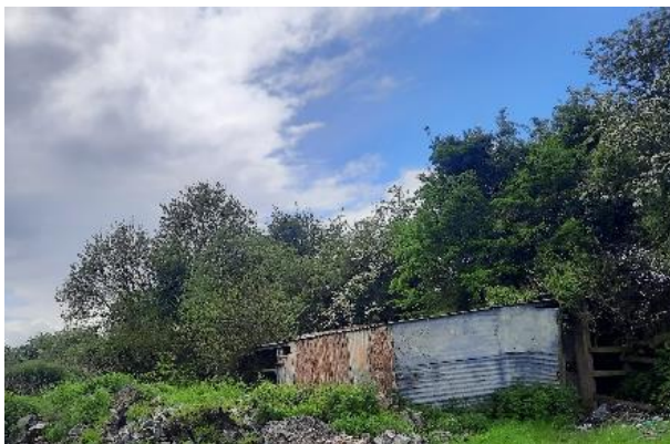
Plate 4-5 Derelict corrugated steel farm shed showing northern facing aspect
