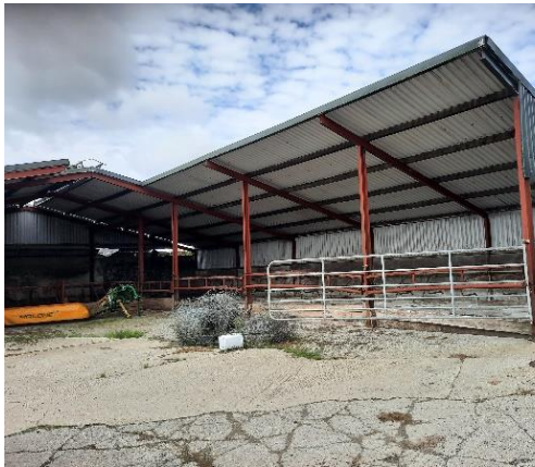
Plate 4-9 Open Slatted shed
