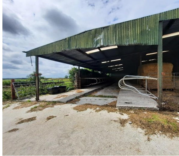
Plate 4-8 Cubicle shed, straw storage and stables
